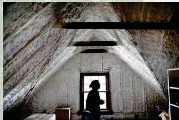
Insulation was sprayed on the attic walls and ceiling.
