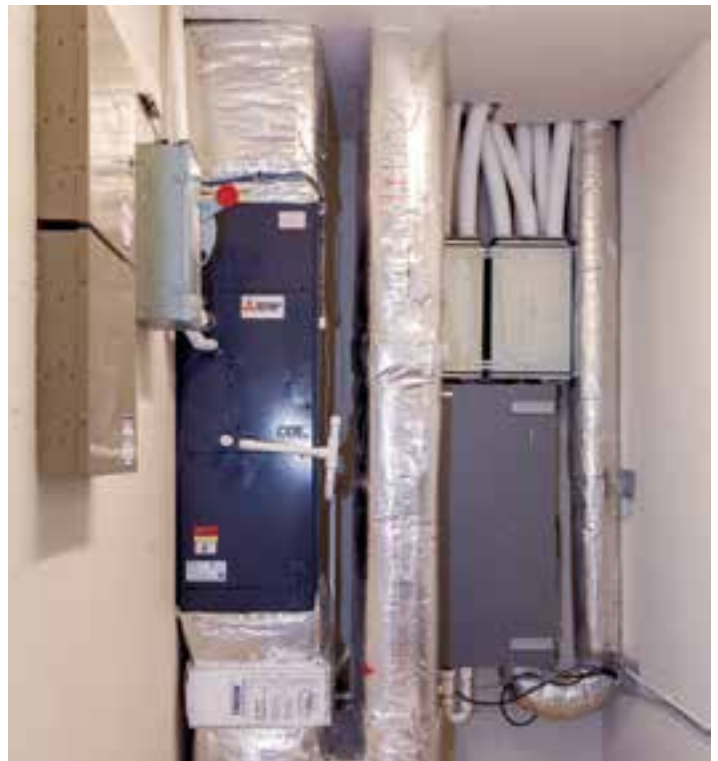
This High-Performance HVAC system supplies fresh air to all rooms while exhausting stale air outside. This system recovers more than 80 percent of the energy contained in the heated and cooled air being exchanged.
