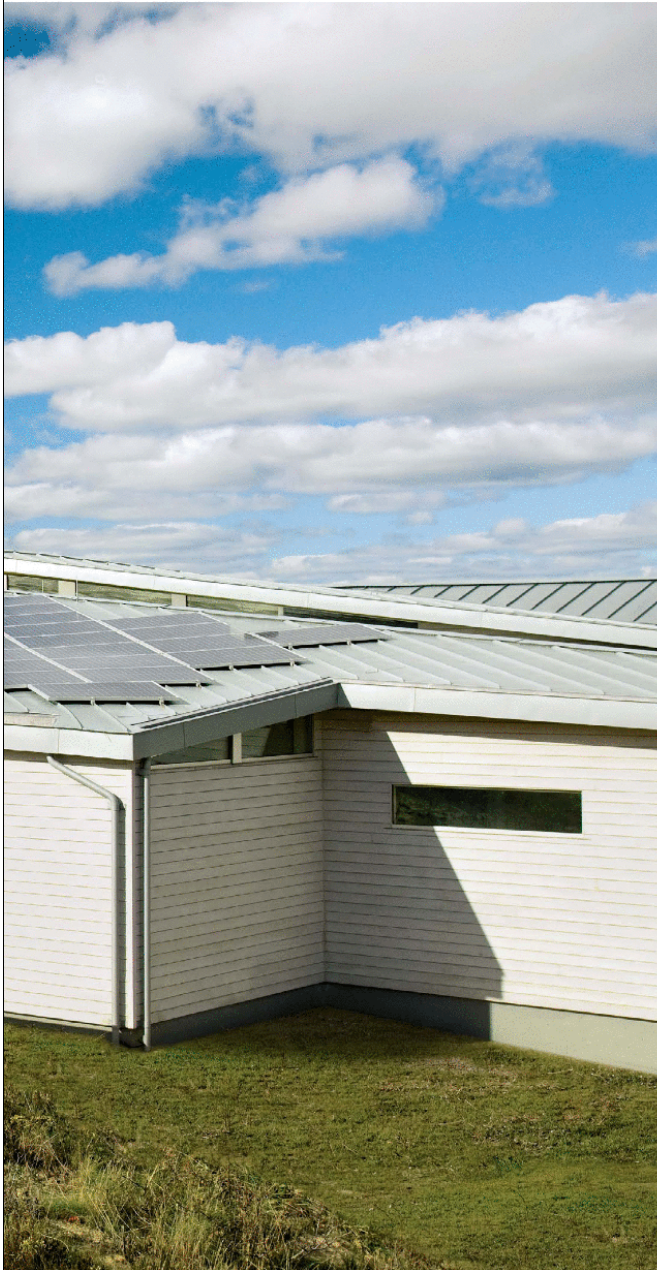
■ THE LOW-KEY ARRAY of photovoltaic panels by Evergreen Solar in Marlborough, Massachusetts, generates electricity for the house, and, in summer, sends excess power to the grid. The roof itself is made of seamed zinc. The narrow windows that slice the shiplap cedar siding on the side and rear facade of the building belie the expansive glass found on the waterview side.
